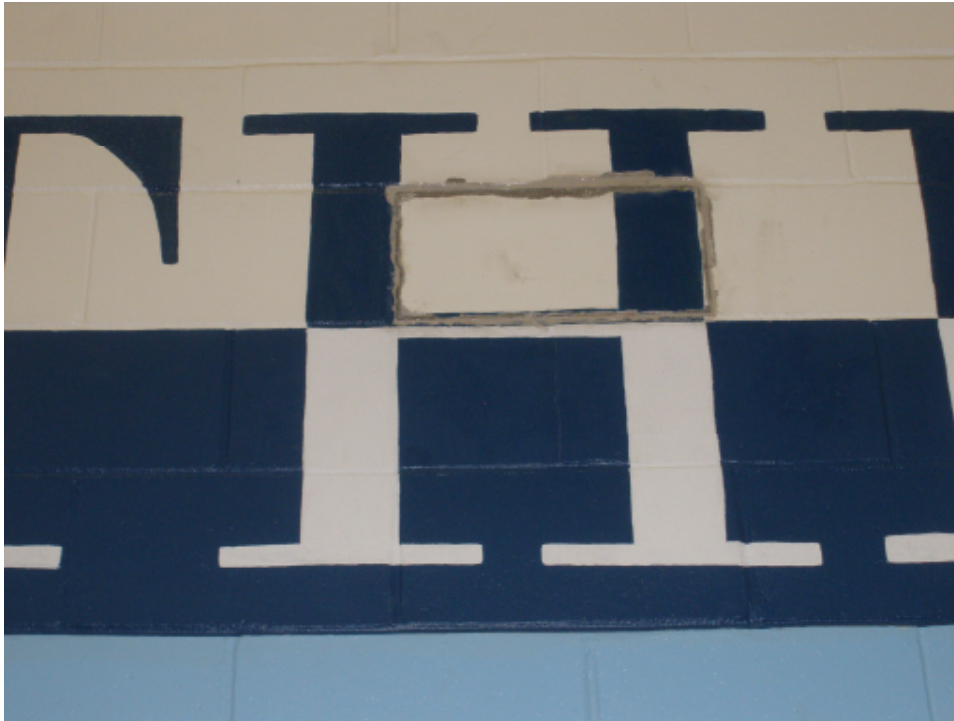
Photo 4: CMU repair over entry portal, S wall of gym.
