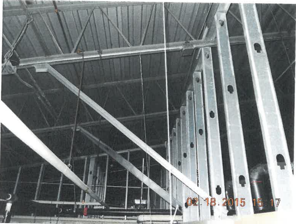
Wall studs and tack connect to roof joist.
