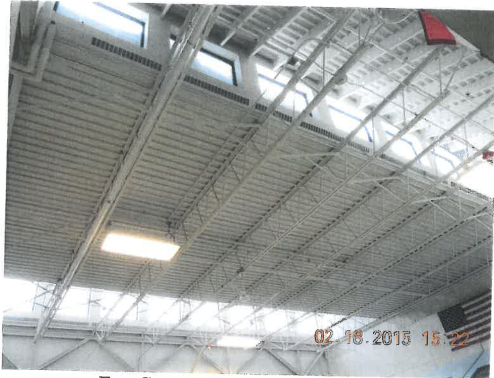
East Commons - roof joists exhibited and measured no significant sag.
