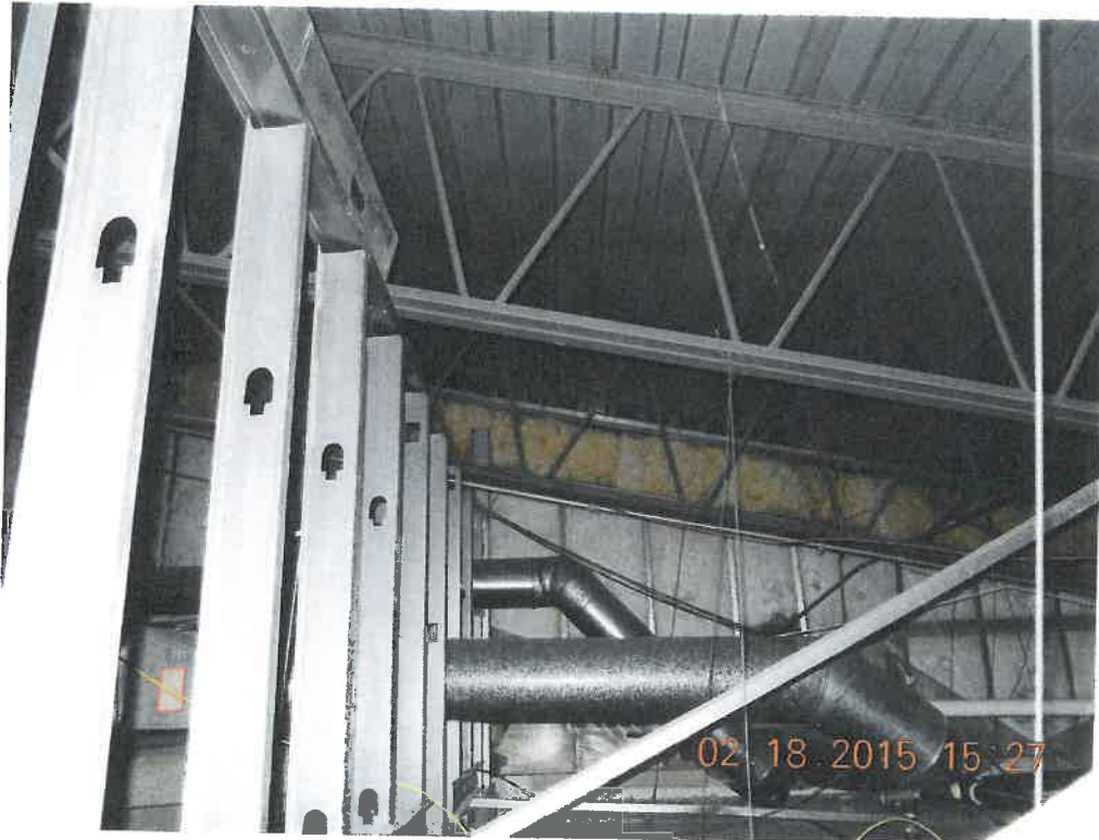
Wall track fastened directly to steel bar joist.
