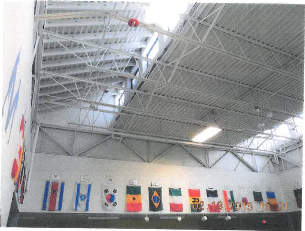
Wall studs and tack connect to roof joist.
