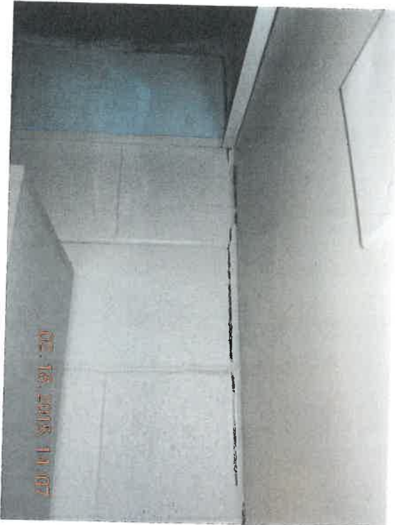
Room 155 - vertical crack at joint of 2 dissimilar walls
