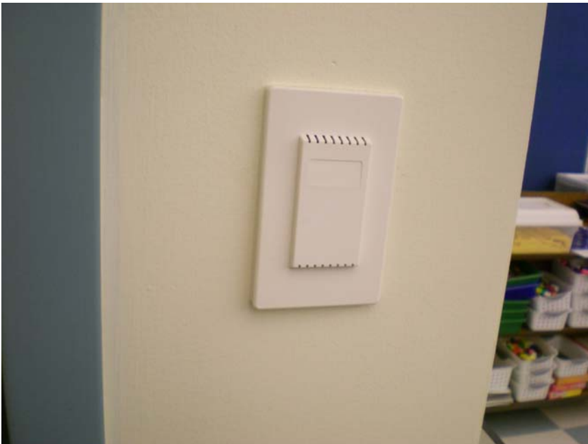
Typical CO2 sensor – mounted on wall
