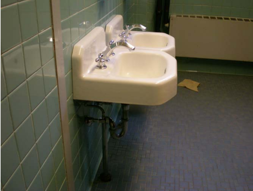
Lavatories at BOYS TOILET 52
