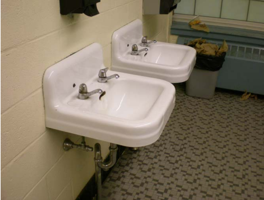
Typical Bathroom Lavatories (age and condition vary throughout the school)
